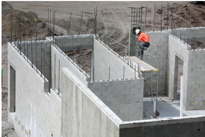
Construction at the Imagine Clearwater site in Clearwater, Fla., in March.
